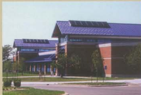
In Kansas City, Casey and Associates converted an abandoned grocery store into a state of the art data center for Jack Henry & Associates of Monett.
